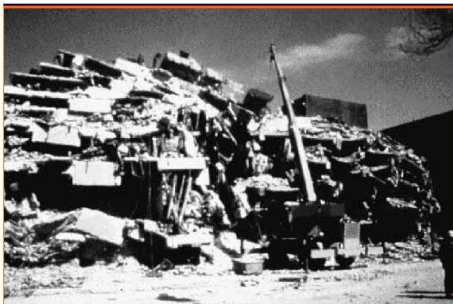
Colapso total del Hospital Juárez (Foto: E.V leyendecker, National Bureau of Standards.)
